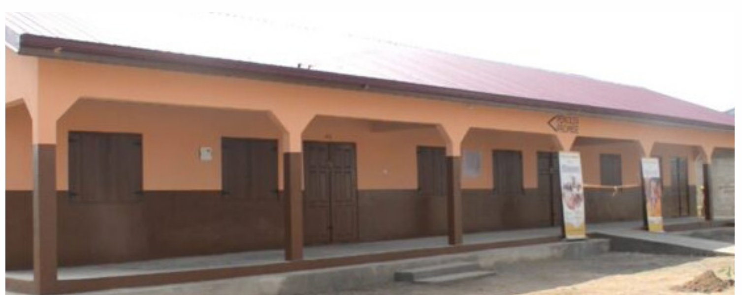
3 unit classroom block
