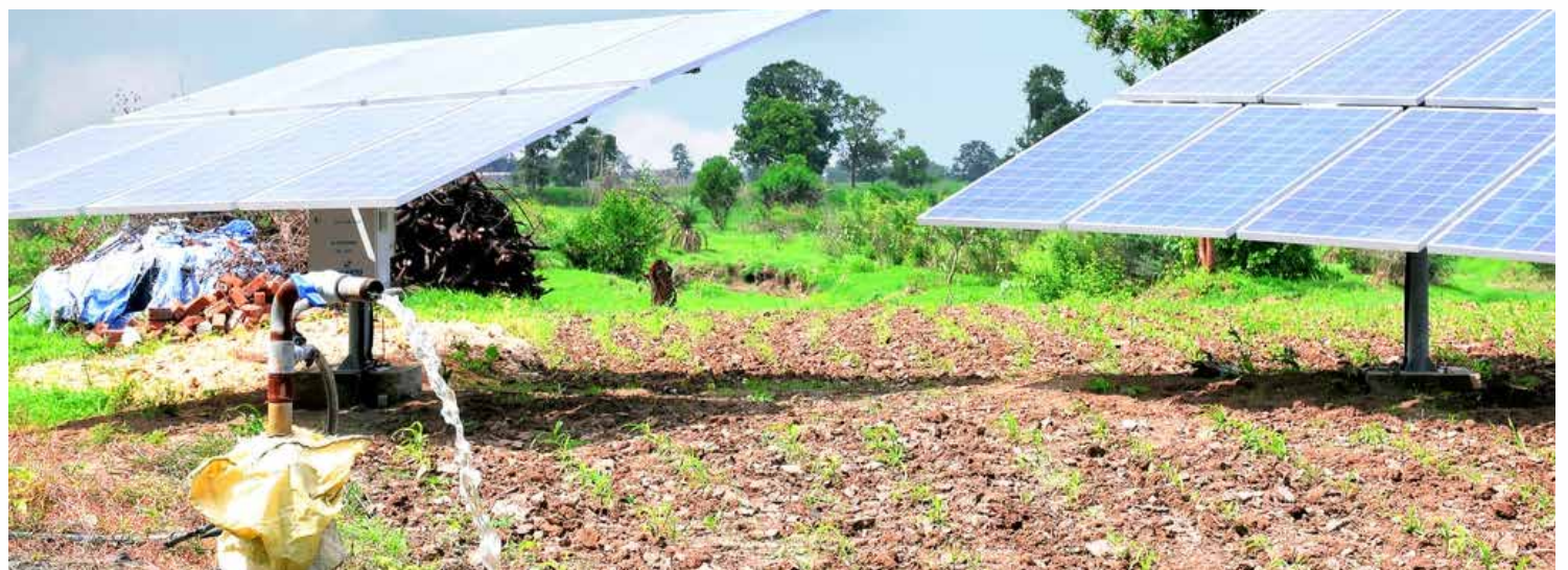
Solar-powered borehole
