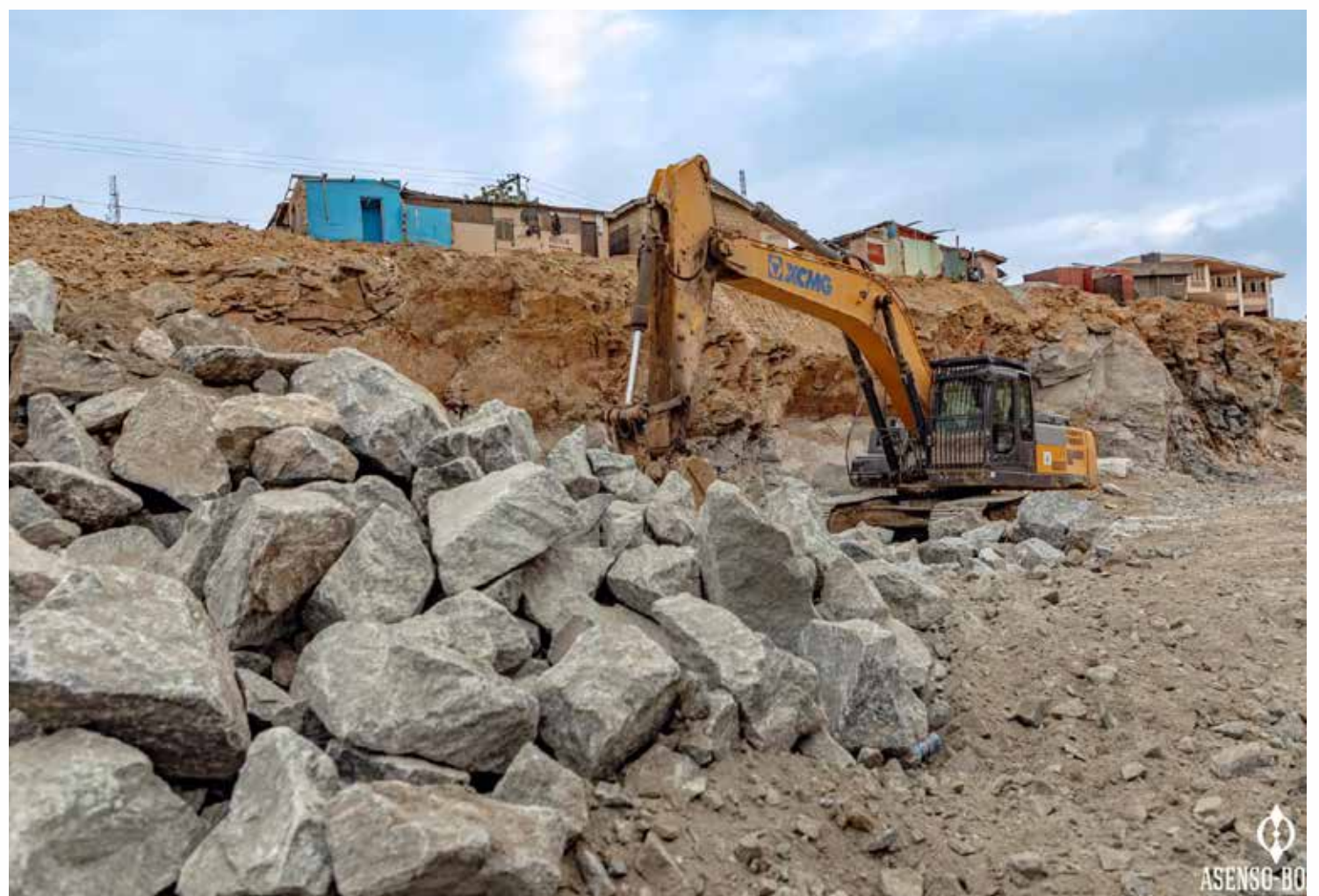
Buduburam road project
