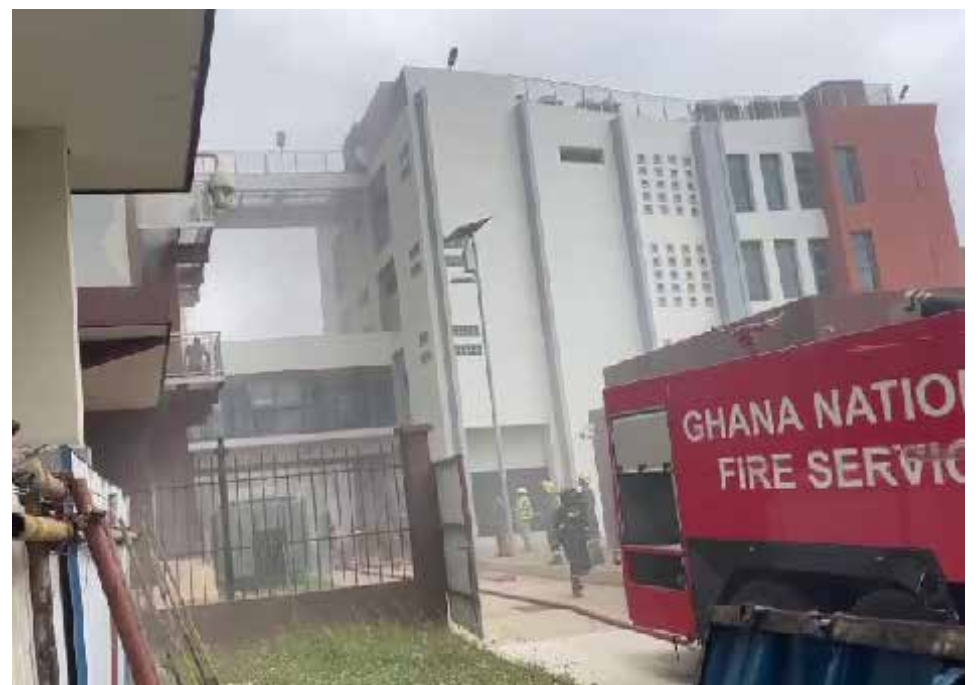
Job 600 Block offices
