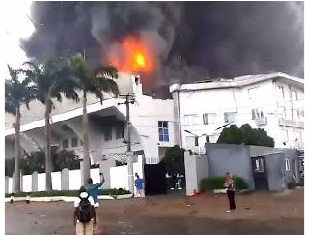
Christ Embassy Headquarters in Lagos on fire
