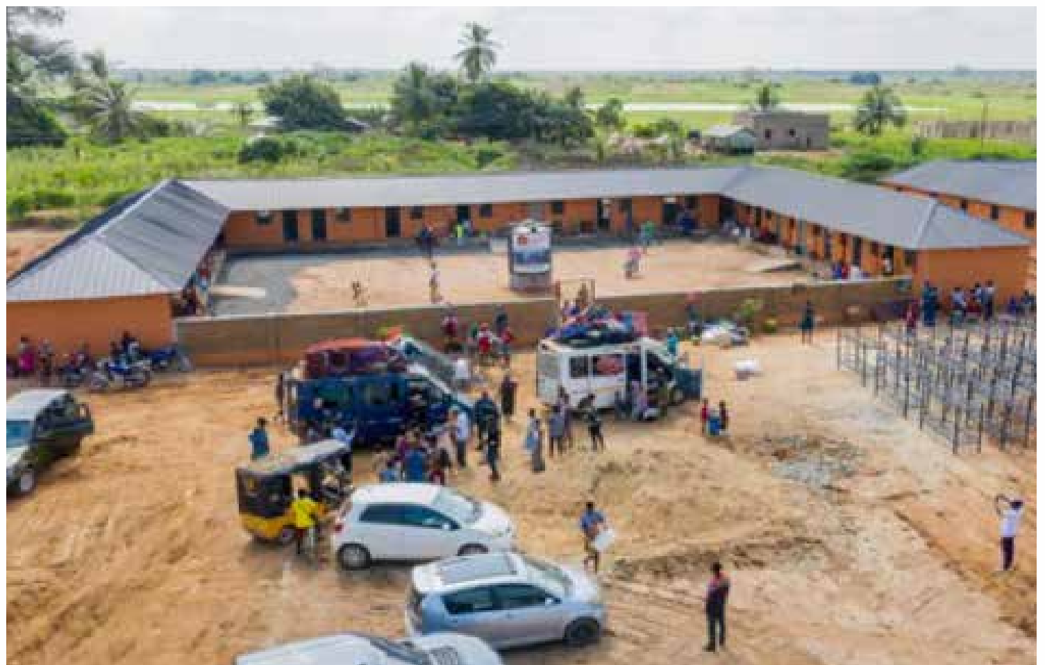
Fully-furnished quarters for 300 Akosombo dam spillage victims
